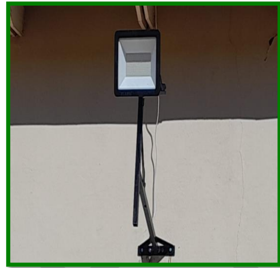
Picture 24: Replacement of door and outside area lighting installed
