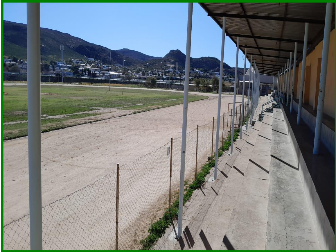
Picture 22: New fencing at sports facility
